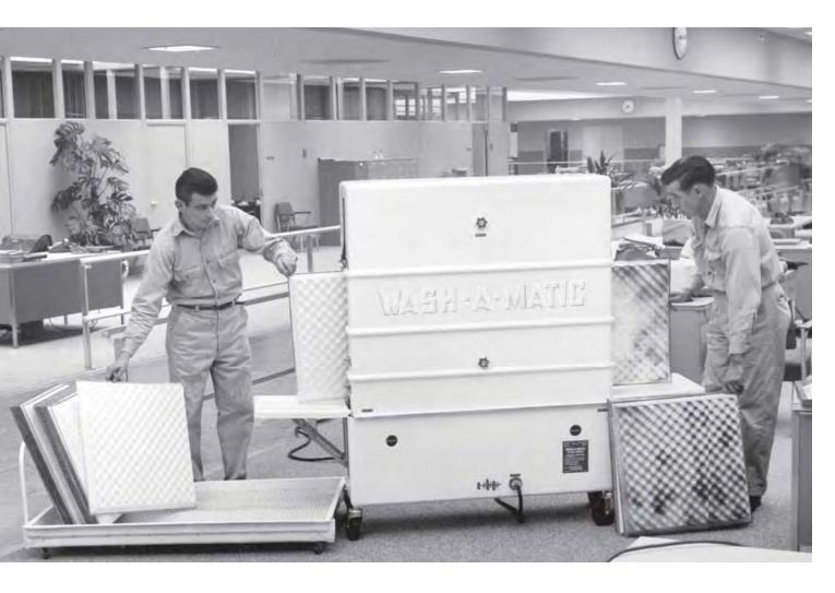
The portable Wash-A-Matic was one of the unusual products distributed by Graybar in the 1960s. It was used to clean ceiling panels.
